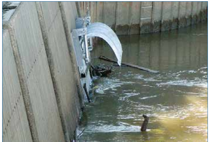
Fig. 66: Screen with automatic cleaning system
