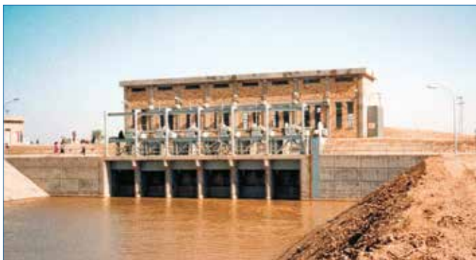
Fig. 3: Building accommodating pumping station
